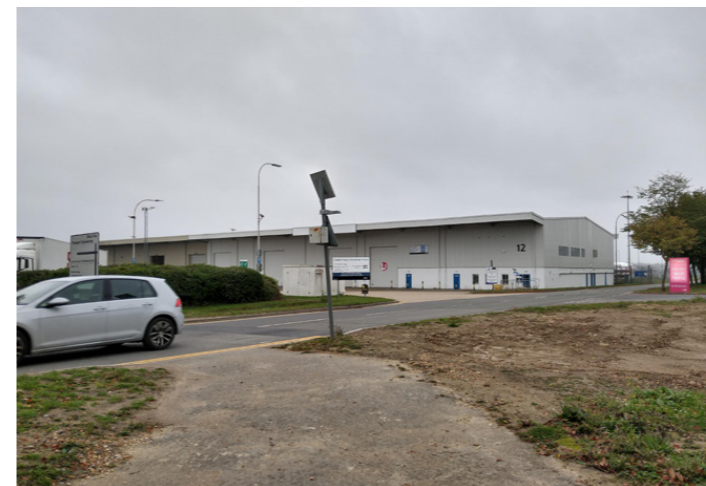
Figure 6. Light Industrial unit on Perimeter Road South
